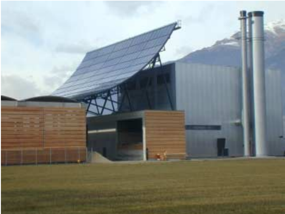
Figure 1: The new biomass CHP plant in Lienz
